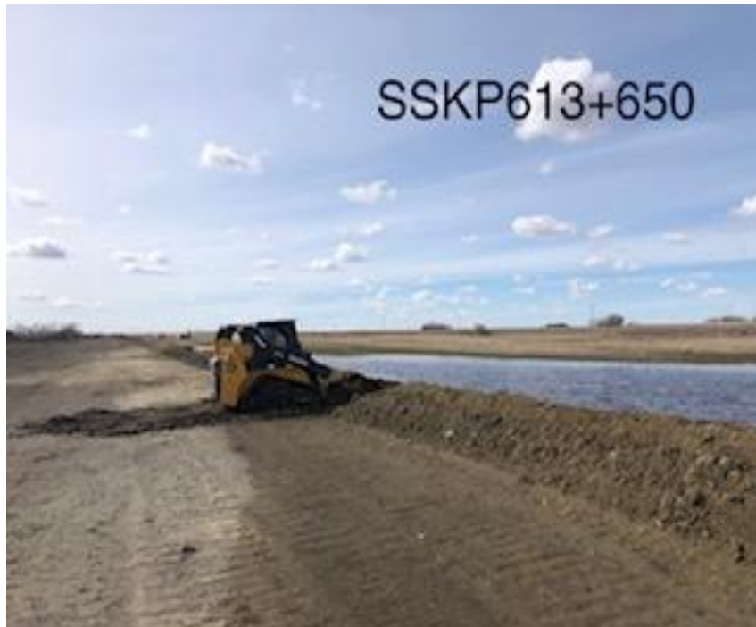
Skid steer used to create a break in roach line to enable the water to dry quicker
