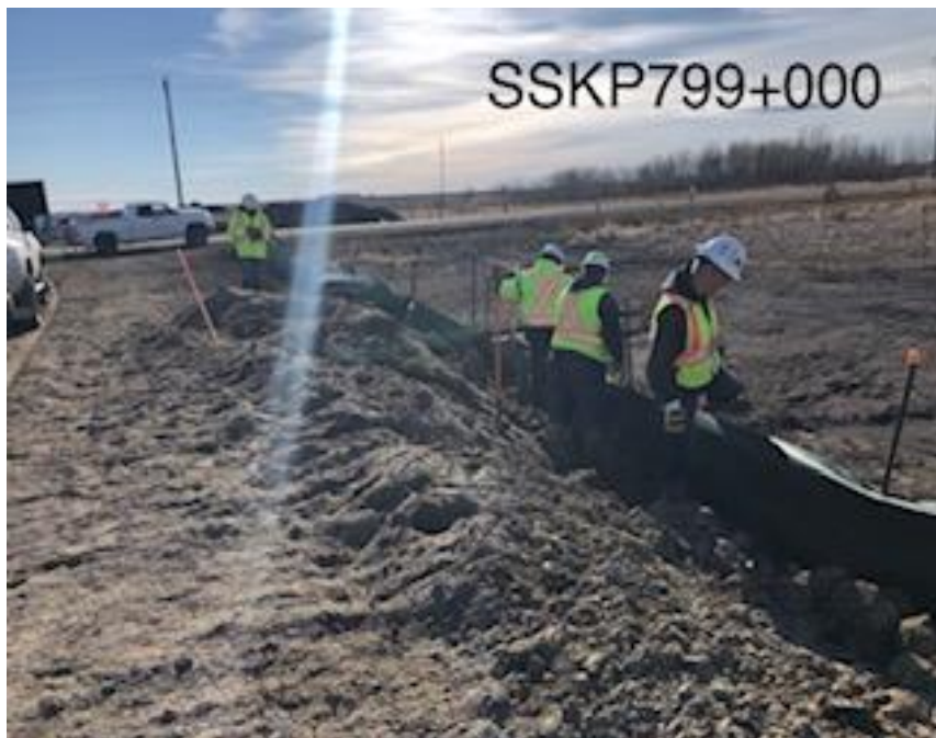
Wing wall that was down was being repaired
