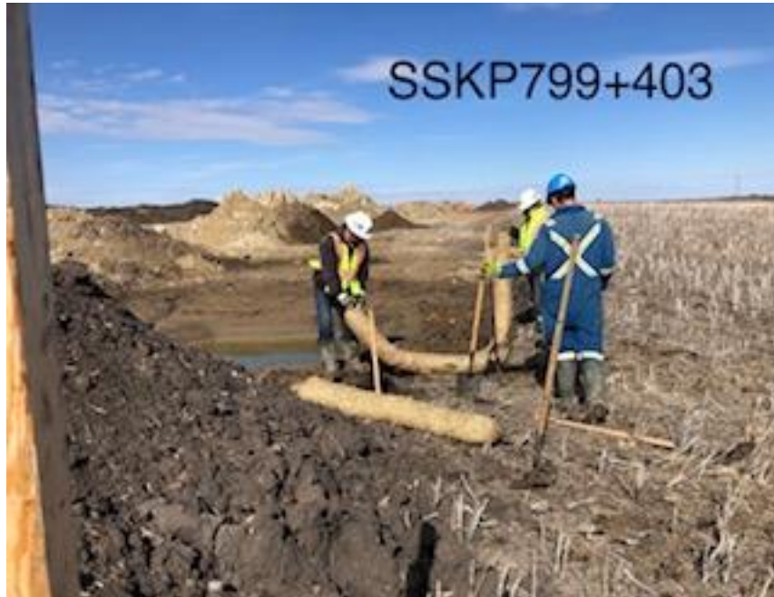
Erosion control devices – straw wattle being installed
